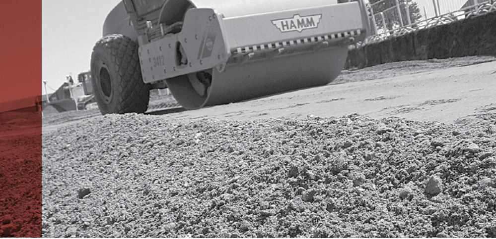
IMAGE 11: Compacting the aggregate fill.
