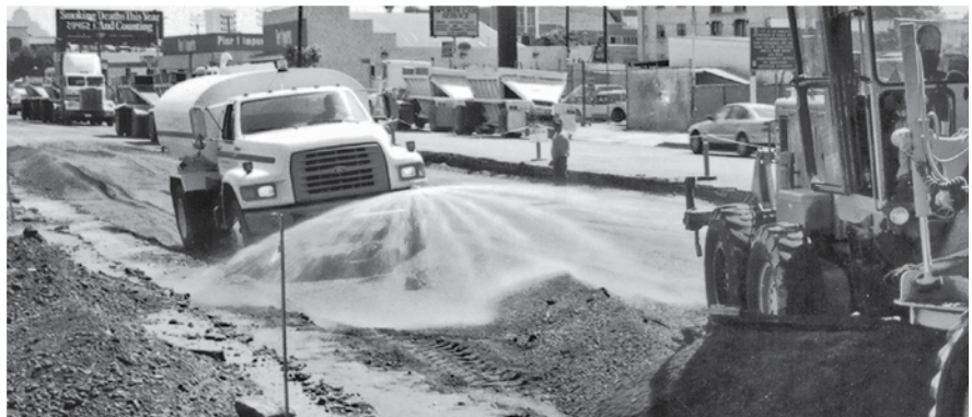
IMAGE 10: Moistening the fill before compaction.
