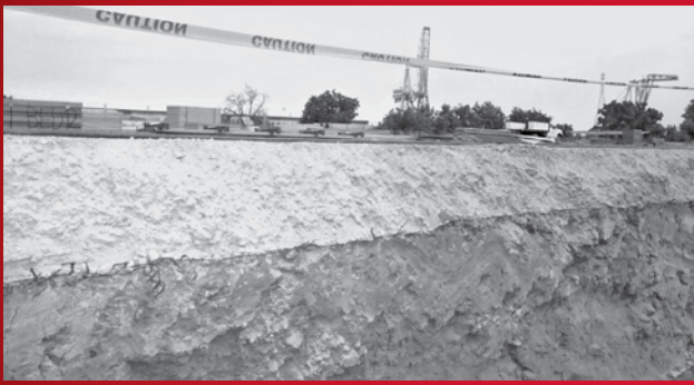
IMAGE 13: A backhoe excavation through Tensar Geogrid.
